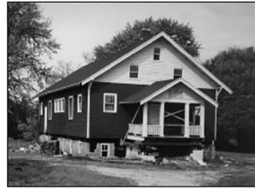
Beaver Valley Grange Hall off the foundation and on jacks.
